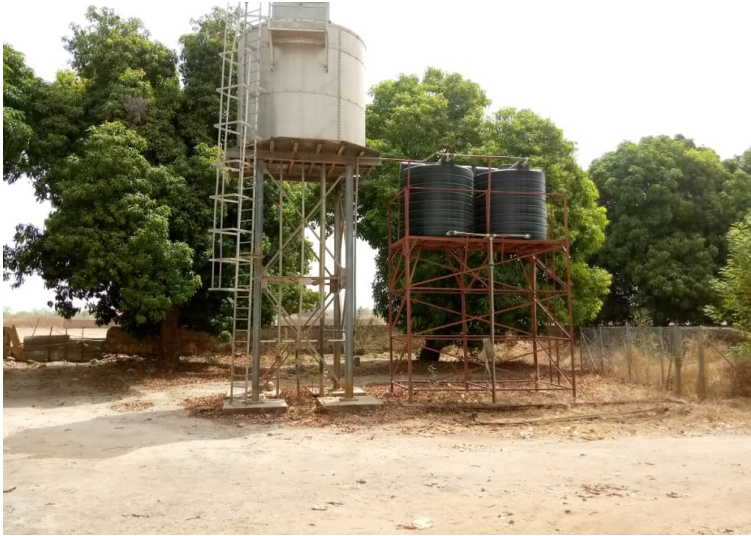
Figure 10: Water tank in TAD TVET Center
