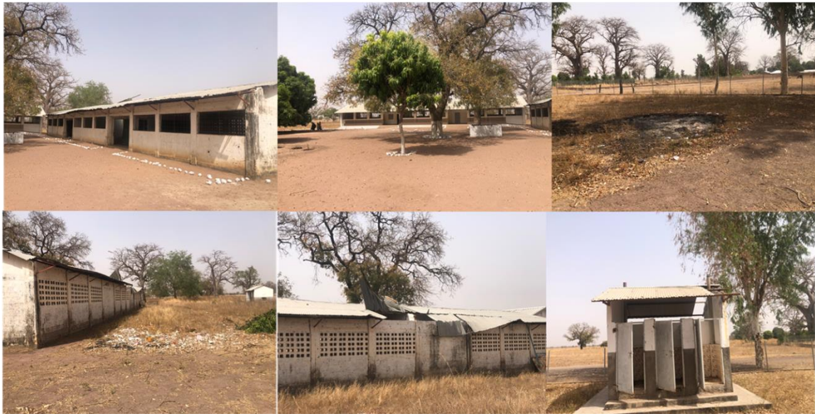
General School Environment and Dilapidated ECD classroom Block and Toilets
